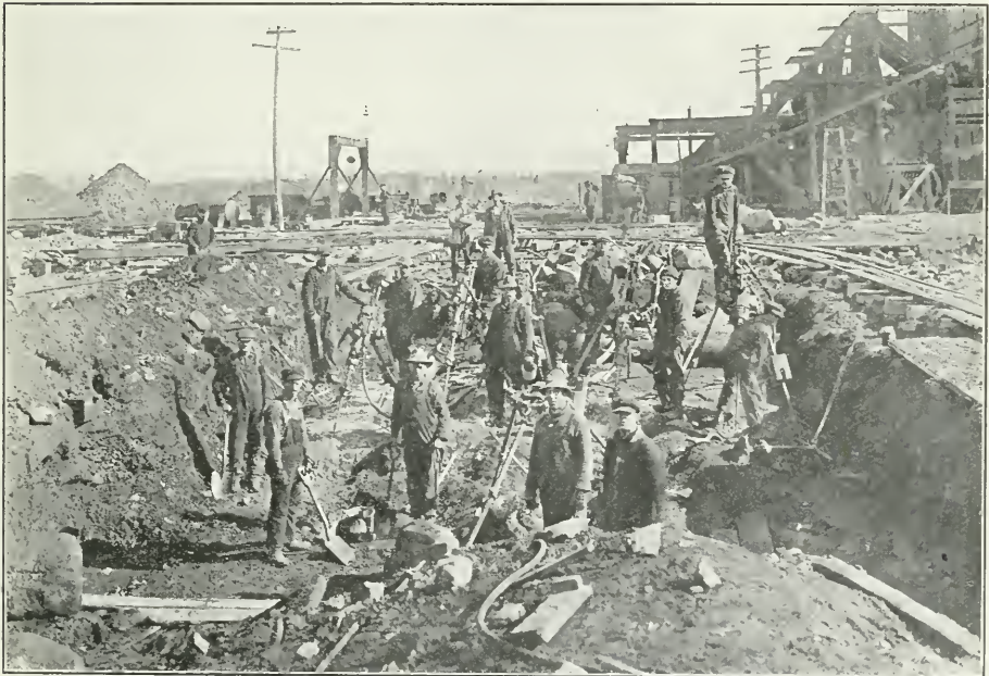
Fig. 66—Commencement of No. 3 shaft, 5 compartments, Creighton mine, 1915.
